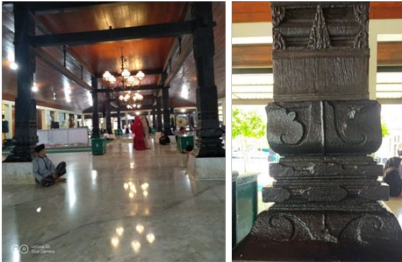
Figure 6 Veranda and Umpak
